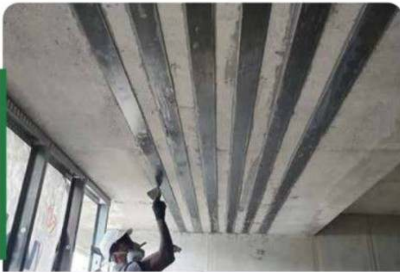
Concrete Repair & Strengthening
